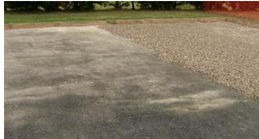
Spreading the top surface over hard base
