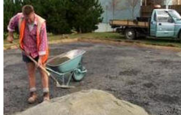
Spreading crushed lime over the base
