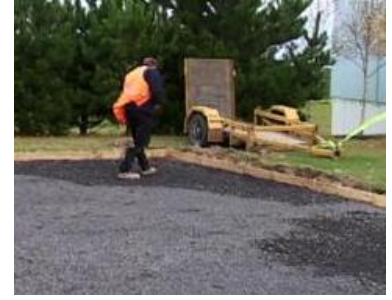
Laying the gravel base
