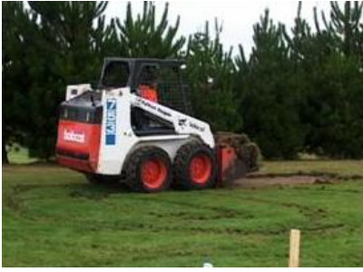
Removing the turf
