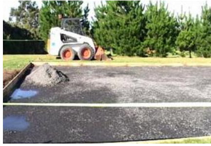
Laying the gravel base
