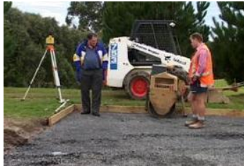
Compacting the base
