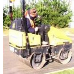
Vibrating roller compacts the crushed lime
